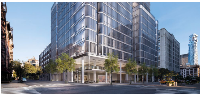
SoHo Tower, New York, USA, 42 spaces, residential
